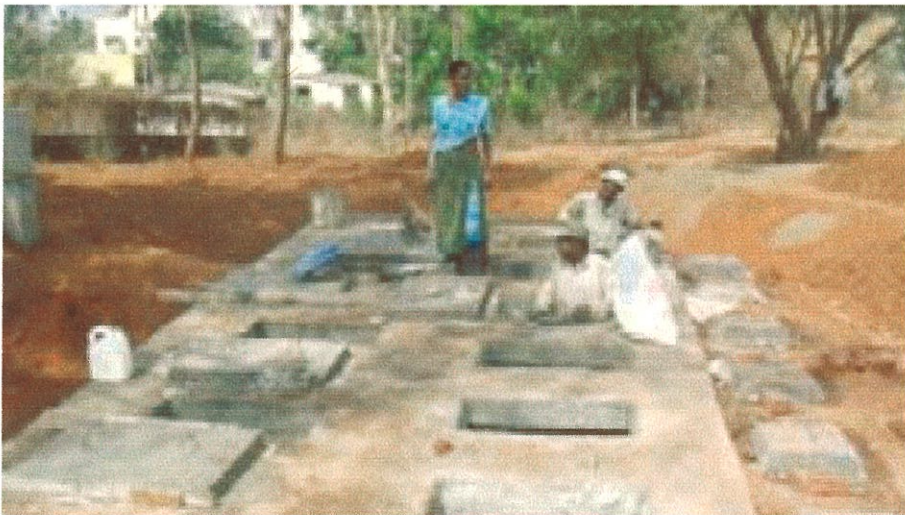
Construction of ABR (r) and AF (l)
