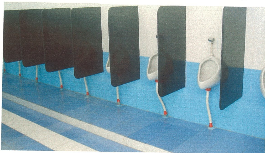
Picture 4: row of waterless urinals in the boys toilet block. (source: ESF, 2008)
