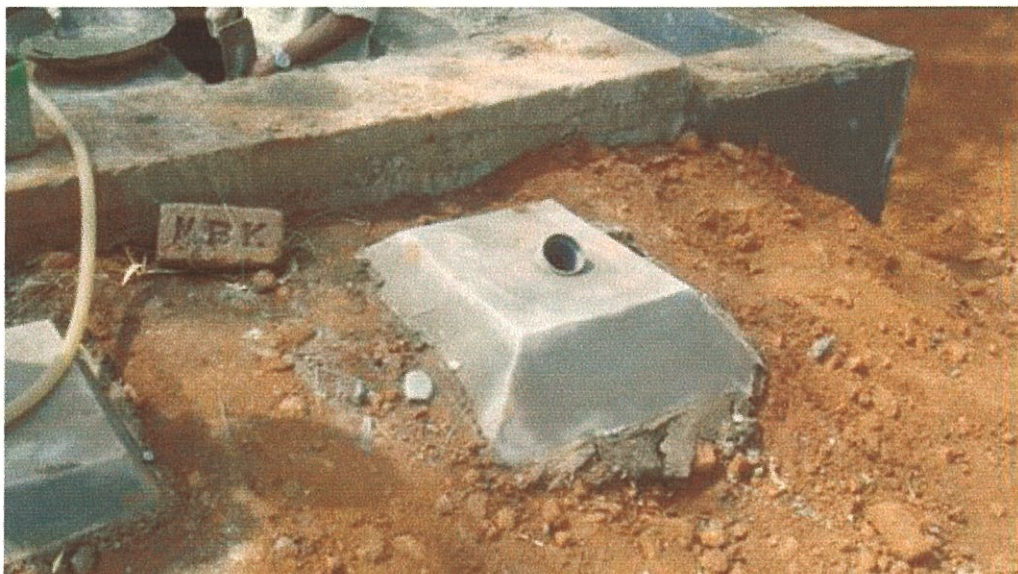
Test pipe into last chamber of the ABR
