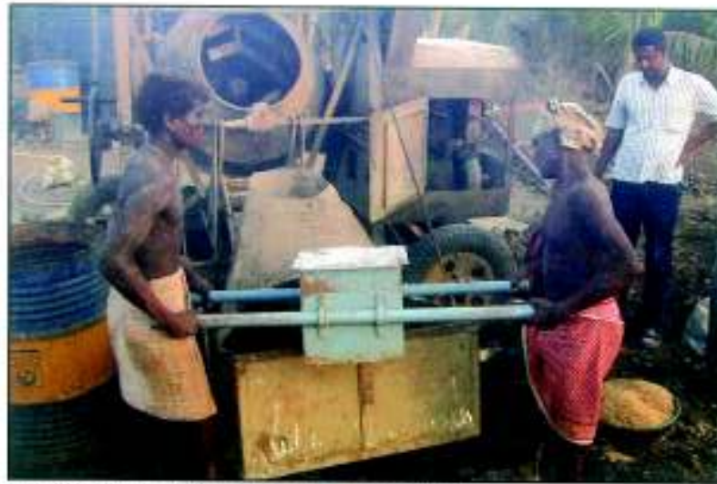
Photo 5.80 : Mixing by mechanical mixer.
