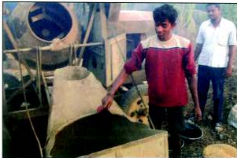
Photo 5.81 : Mixing by mechanical mixer.
