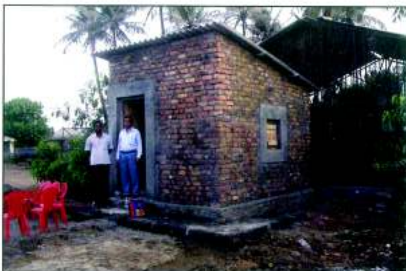
Photo 5.107 : Shed constructed by use of sample bricks.
