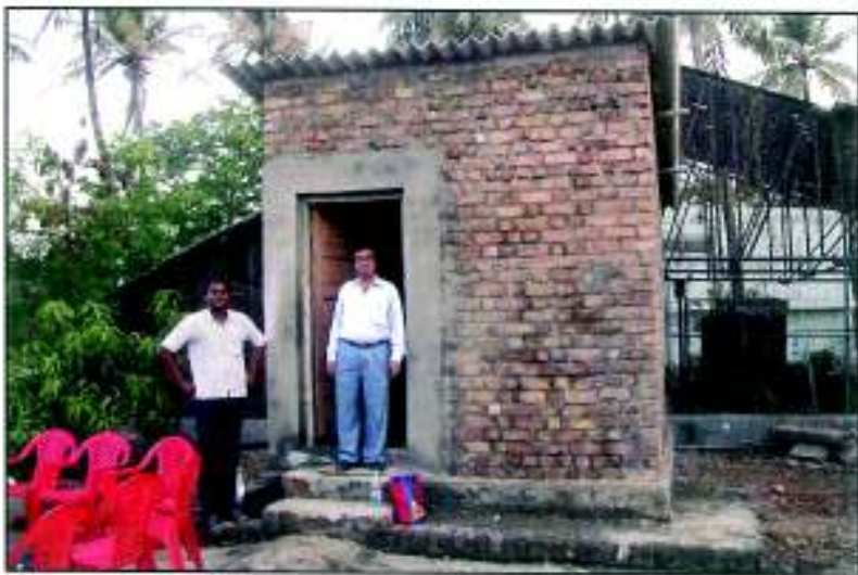
Photo 5.106 : Shed constructed by use of sample bricks.
