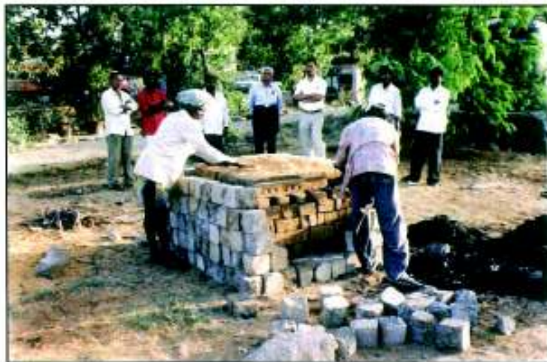
Photo 3.14 : While arranging the kiln.
