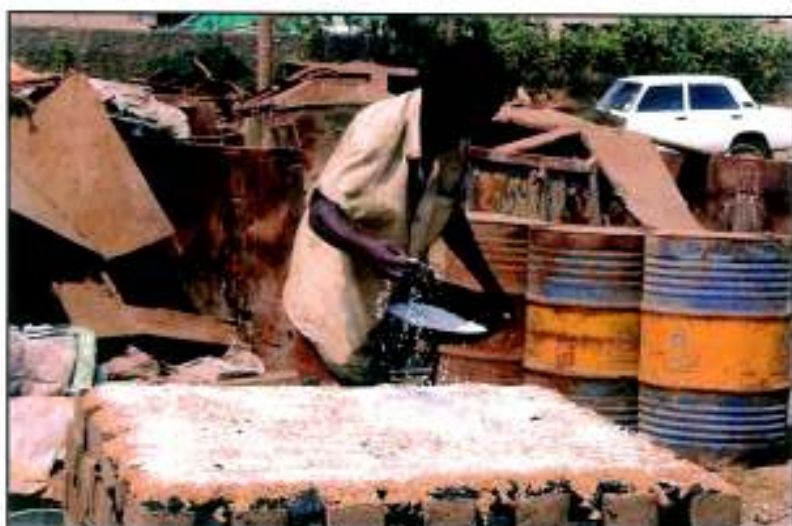
Photo 5.30 : Completing 5th layer of kiln for sample no. 1.
