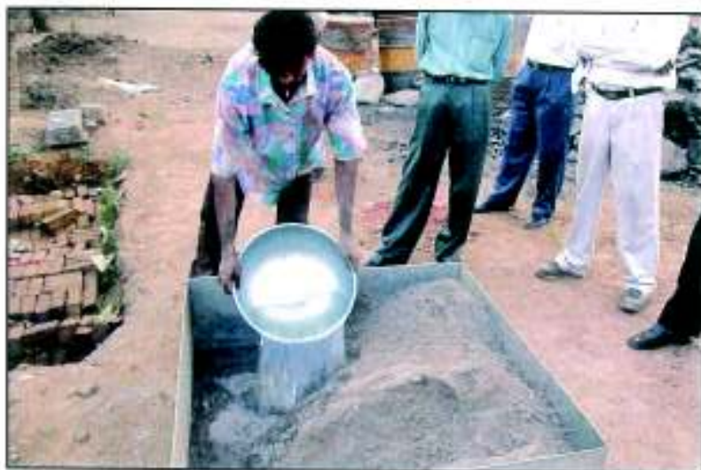
Photo 5.64 : Adding water in dry mix.
