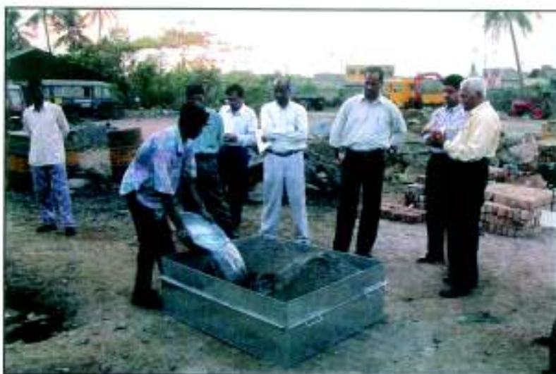
Photo 5.65 : Adding water in dry mix.
