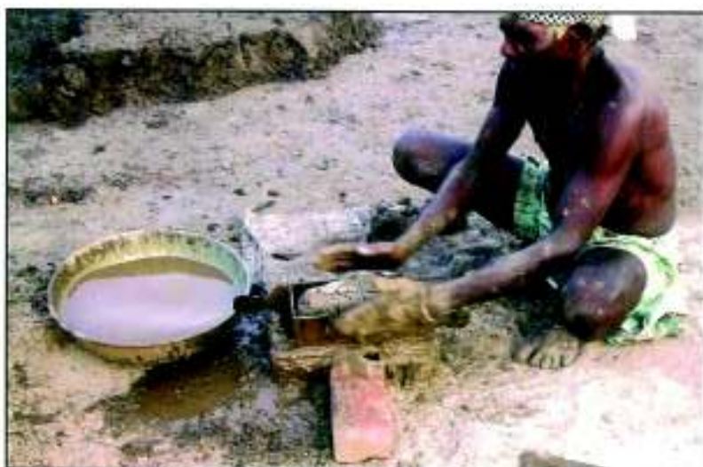
Photo 5.90 : Moulding of bricks.
