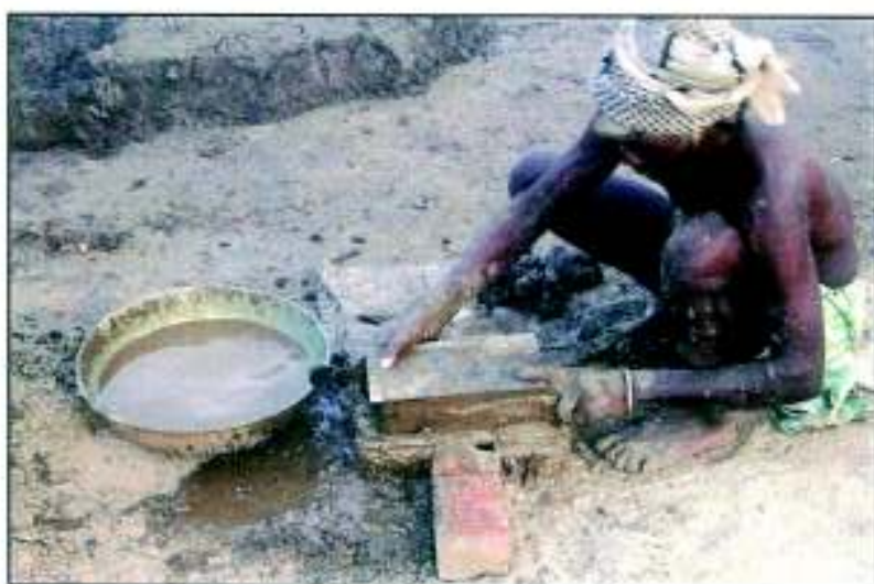
Photo 5.3 : While moulding the bricks.
