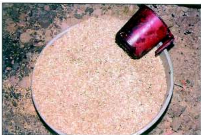
Photo 5.88 : Adding paddy foilage to mix.
