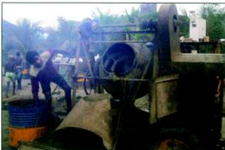
Photo 5.83 : Adding water to mix.
