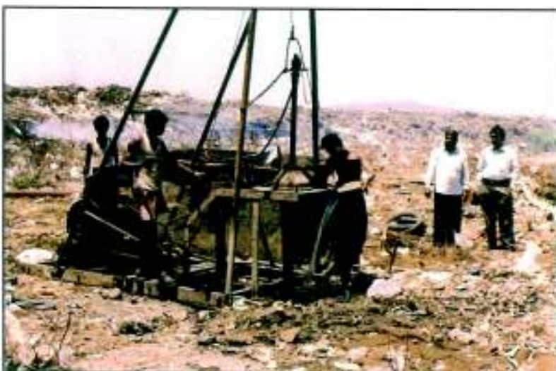
Photo 4.14 : While taking the trial bores.
