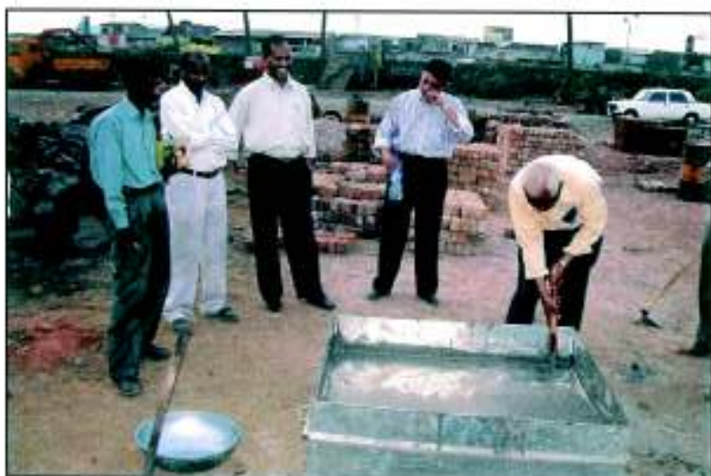
Photo 5.70 : Inspection of wet mix.
