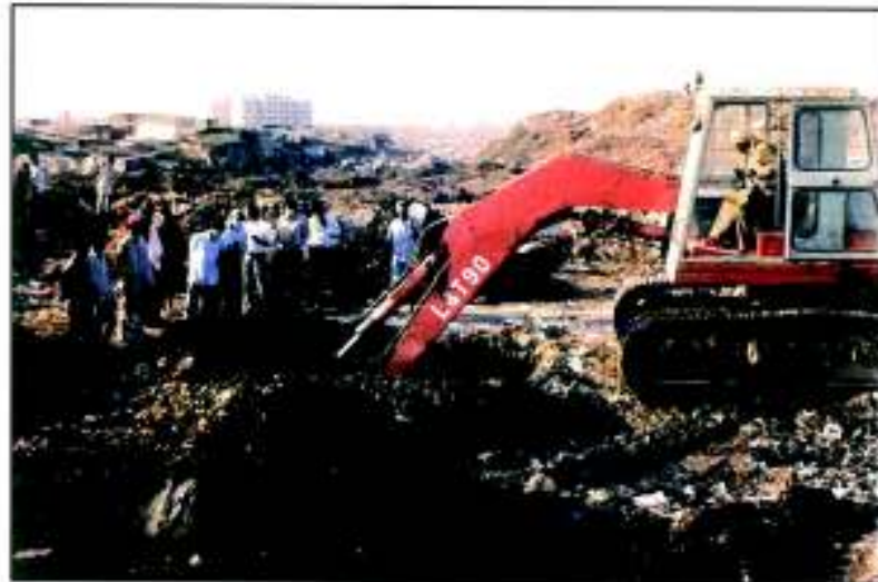
Photo 4.5 : While excavating trial pit.
