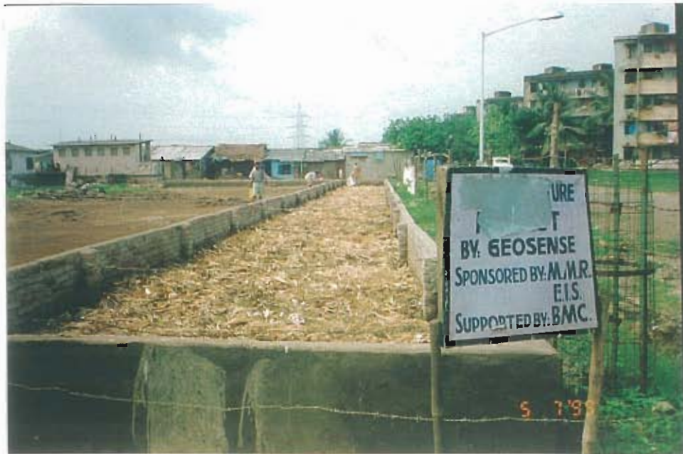
Plate 5: 'Constructed' bin-with brick walls to acquire necessary depth - in operation.
