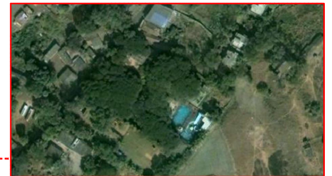
Pavan resort at akloli with swimming pools and water park. This emerging typology of resorts is of concern as, their large paved areas and gardens if unregulated increase runoff and erosion.
